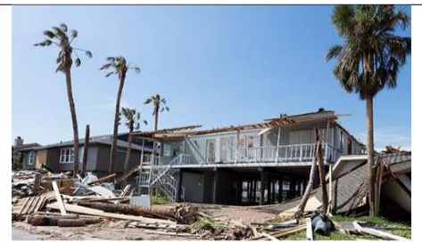
Strong wind damages buildings
